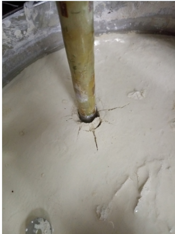
Fig. 4. Development of a gap around the pile in the soft clay
